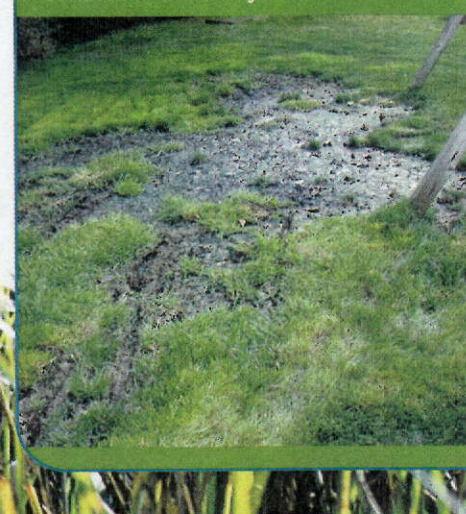
Effluent from a failed drainfield has surfaced in this backyard.
